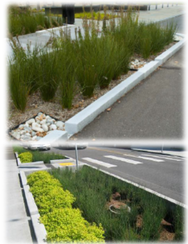
Bioswales and storm water planters: Example of green infrastructure that may be incorporated in future projects, OHM Engineering
