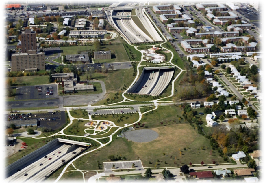
I-696 Bridge Decks aerial photo
