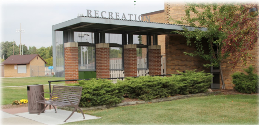
Oak Park Community Center, Recreation entrance
