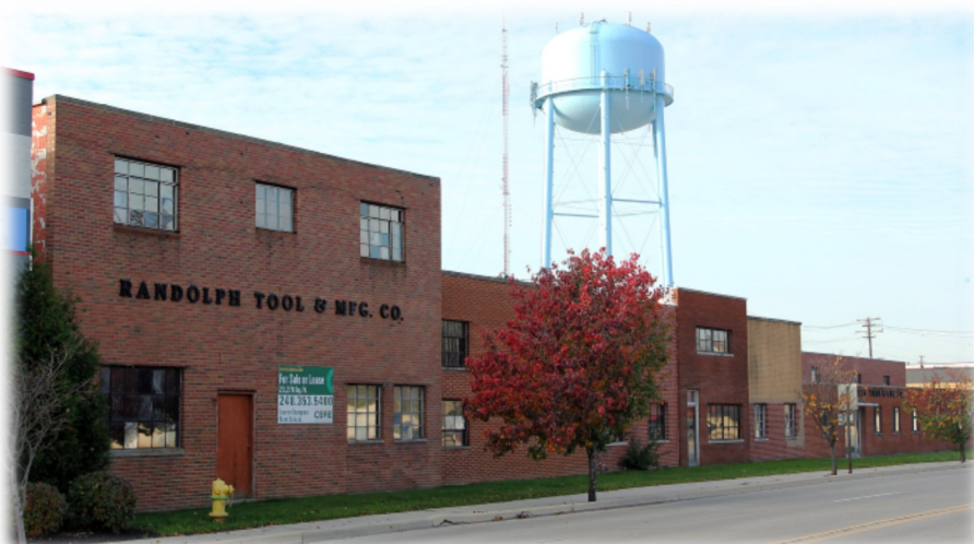
Randolph Tool Building on Eleven Mile, prime redevelopment for Brewpub
