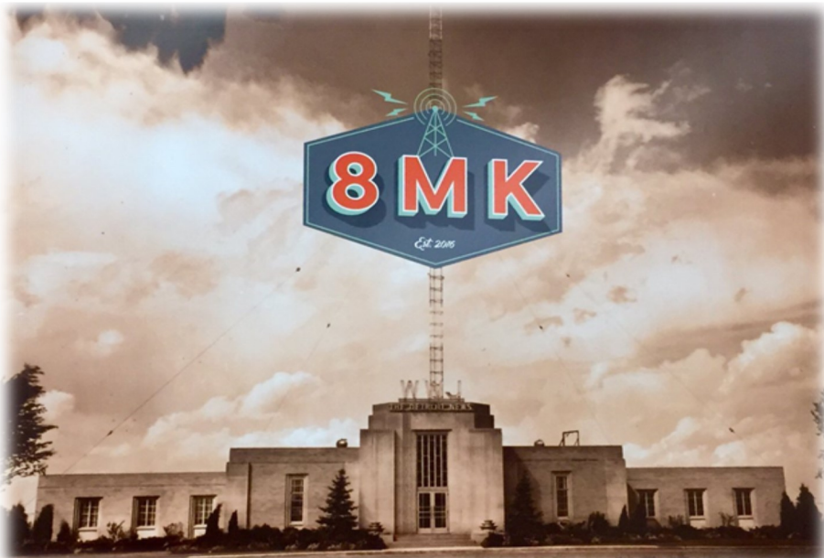
WWJ building, scheduled to be rehabilitated and repurposed into a restaurant
