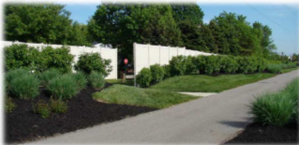
Example of consistent screening along greenbelts, OHM Engineering
