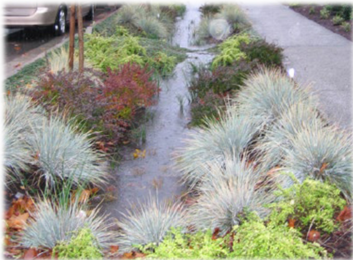
Rain Garden: Example of green infrastructure that may be incorporated in future projects, OHM Engineering
